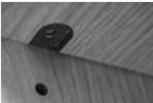
Adjustment holes and secured inset shelf clip
