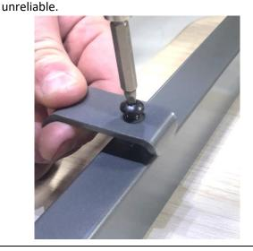
2. Drill a pilot hole in the marked location using a 1/8" diameter drill bit. This will ensure that the self-drilling screw goes in easily and in the correct location. Be sure clean up all metal shavings to prevent injury or damage to other products.
